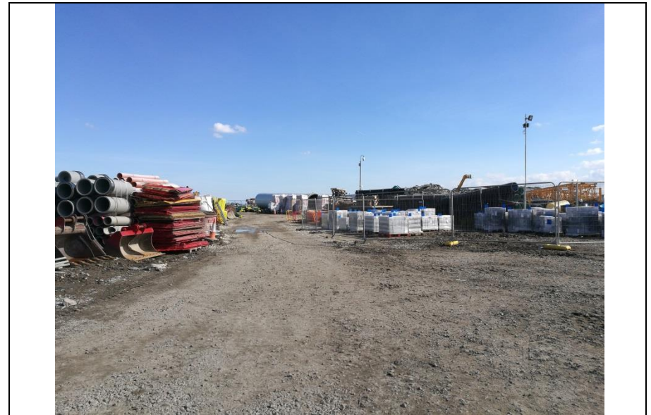
Photo 4 - General view of K3 construction laydown area
