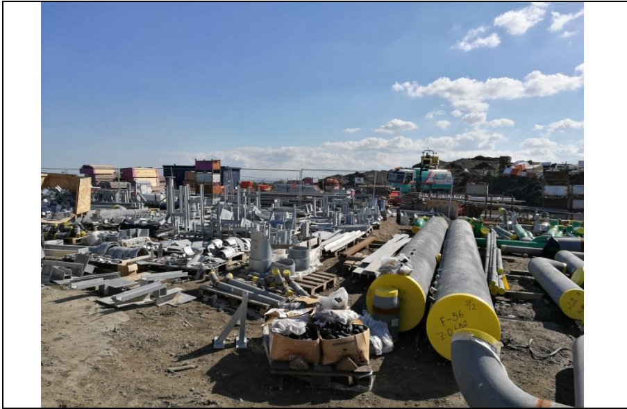
Photo 1 - General view of K3 construction laydown area
