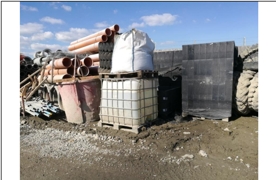
Photo 3 - IBC on northern boundary
